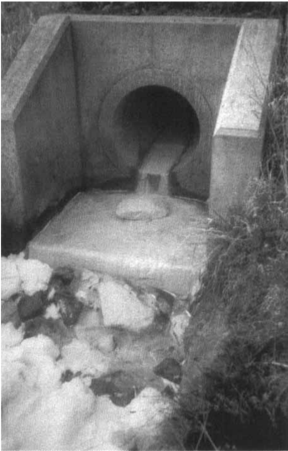
Fig. 2. Culvert at Morrison Busty colliery (before commencement of study) showing deposits of ‘alum’
